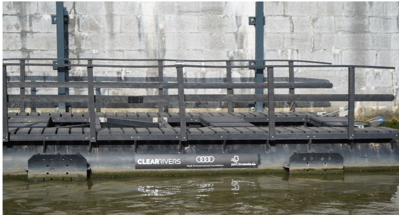
Figure 26: three years old Litter Trap LT6 in Belgium
